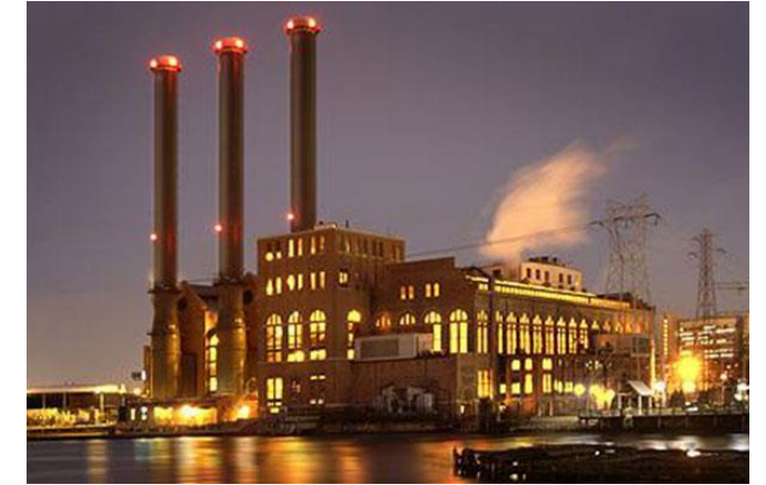
Manchester Street Power Station, Providence
