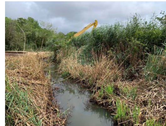
Removal of phragmites within Buckeye Brook to improve ecological health of the stream and increase water-holding capacity for flood reduction, funded by NPS Section 319 Grants (RIDEM)
