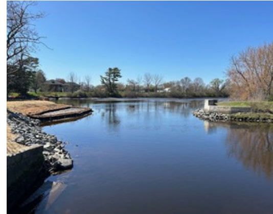
Removal of the Upper and Lower Kickemuit Dams was supported through the Climate Resilience Fund (RIDEM)
