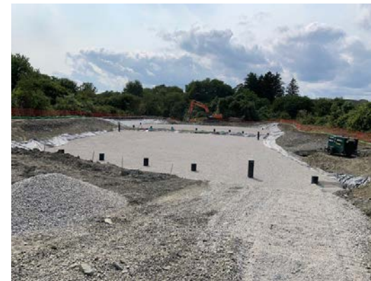
Installation of a wet vegetated treatment system (WVTS) in Middletown funded by NPS Section 319 Grants (RIDEM)
