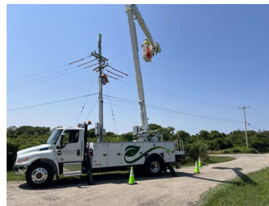
Grid modernization in progress (OER)
