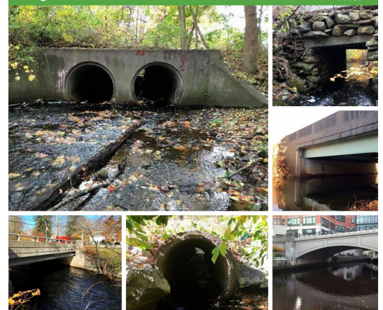
RIDOT's Road-Stream Crossing Design Manual, to be used in conjunction with the RIDOT Road-Stream Crossing Assessment Handbook. Photo courtesy of RIDOT.
