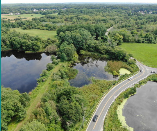
Schoolhouse Road reservoir causeway crossing. The Upper Kickemuit River Dam is the earthen structure to the left of the roadway. Photo courtesy of RIDOT.
