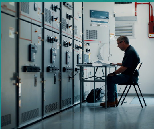
The new Pascoag Utility District Energy Storage System can contribute 650 MWh annually - roughly a quarter of PUD's peak load. Photo courtesy of RIB.
