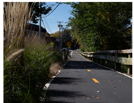
San Souci Bikeway, which connects the Woonasquatucket River and Olneyville Square. This project was financed through the Stormwater Project Accelerator. Photo courtesy of RIIB.
