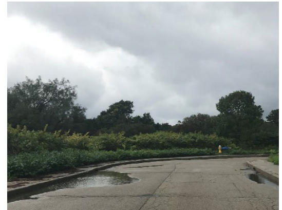
A portion of Spouting Rock Drive that will be removed to expand the drainage buffer around Almy Pond in Newport. Photo courtesy of City of Newport.
