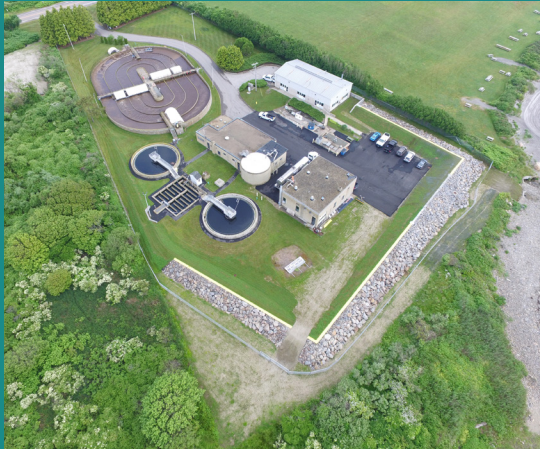
Improvements at Scarborough Wastewater Treatment Facility will reduce future flooding at the facility. Photo courtesy of Town of Narragansett.
